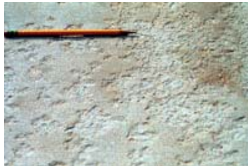
Figure 2-1: Surface scaling of concrete
